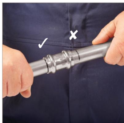
To assemble the joint, the tube must be inserted into the fitting up to the tube stop. (Use the mark on the tube which was made earlier as reference). The pressing operation should only be undertaken when the tube reaches the tube stop (see section 8).
