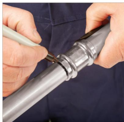
The tube must be fully inserted into the fitting until it reaches the tube stop in order to make a perfect joint. Marking insertion depth will ensure that any tube movement is detected, which is especially important if the joints are to be pressed at a later time.
