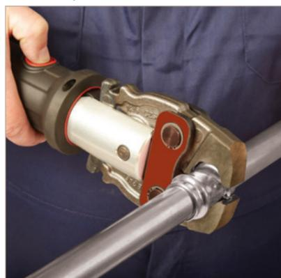
Ensure that the correct size jaw for the fitting is inserted into the tool. The jaws must be placed square on the fitting. Depress the trigger/button to begin the compression cycle of the tool. This is complete when the mouth of the fitting is fully enclosed by the jaws. Now release the jaws from around the fitting. (For further information refer to tooling instructions).
